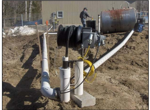
Figure 3. Free-product recovery system
