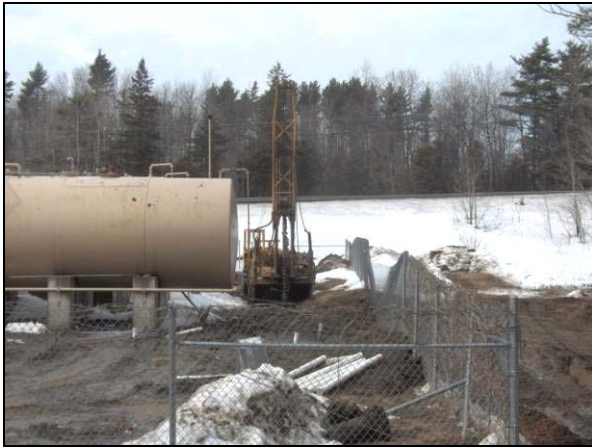
Figure 1. Installation of recovery wells during the initial spill response.
