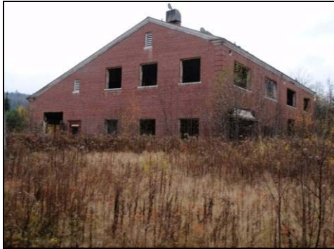
Figure 1. Former Pump House
